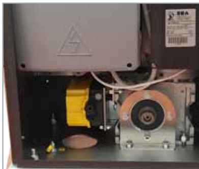
Internal view - Internal photo
