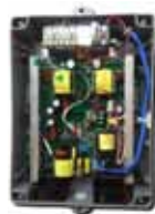
Battery back up with fan cooling systems
